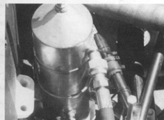
Tank installed, showing routing of oil hoses
